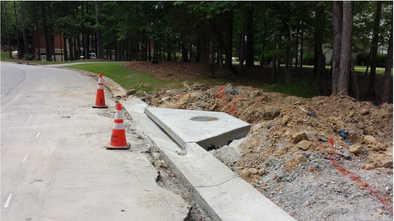
Photo 1: New catch basin lids are complete. (05/12/2015)
