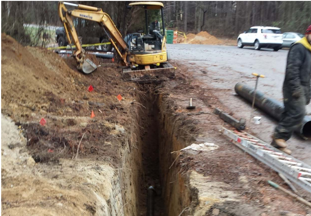
Photo 1: Utility relocation underway. (01/14/2015)
