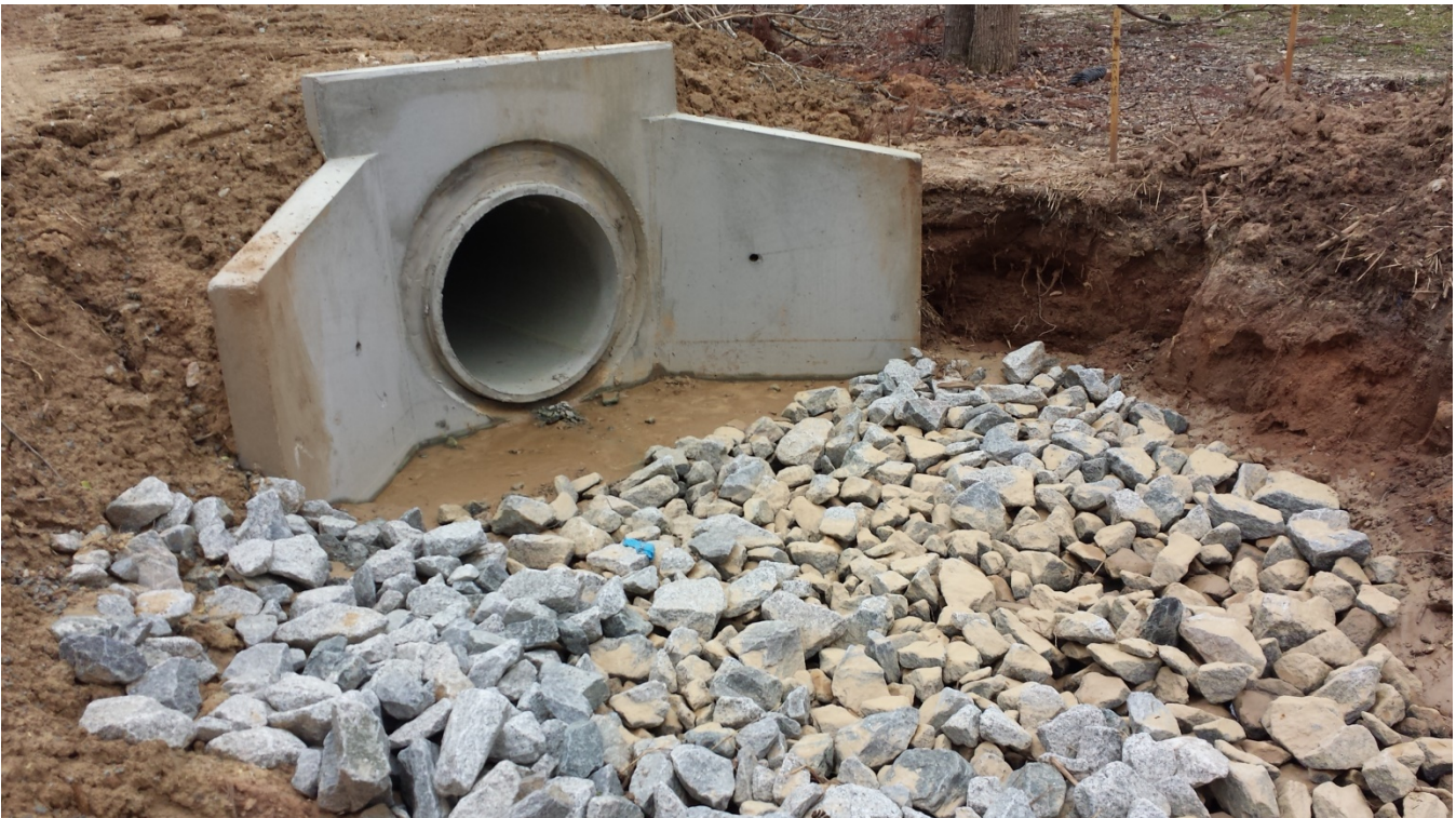
Photo 2: Rip rap has been placed at the outlet side of pipe.
