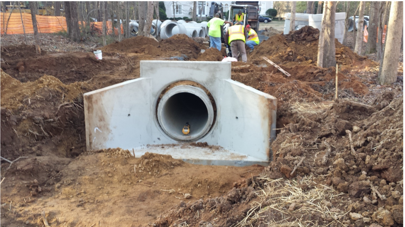
Photo 2: New concreted headwall installation in progress.
