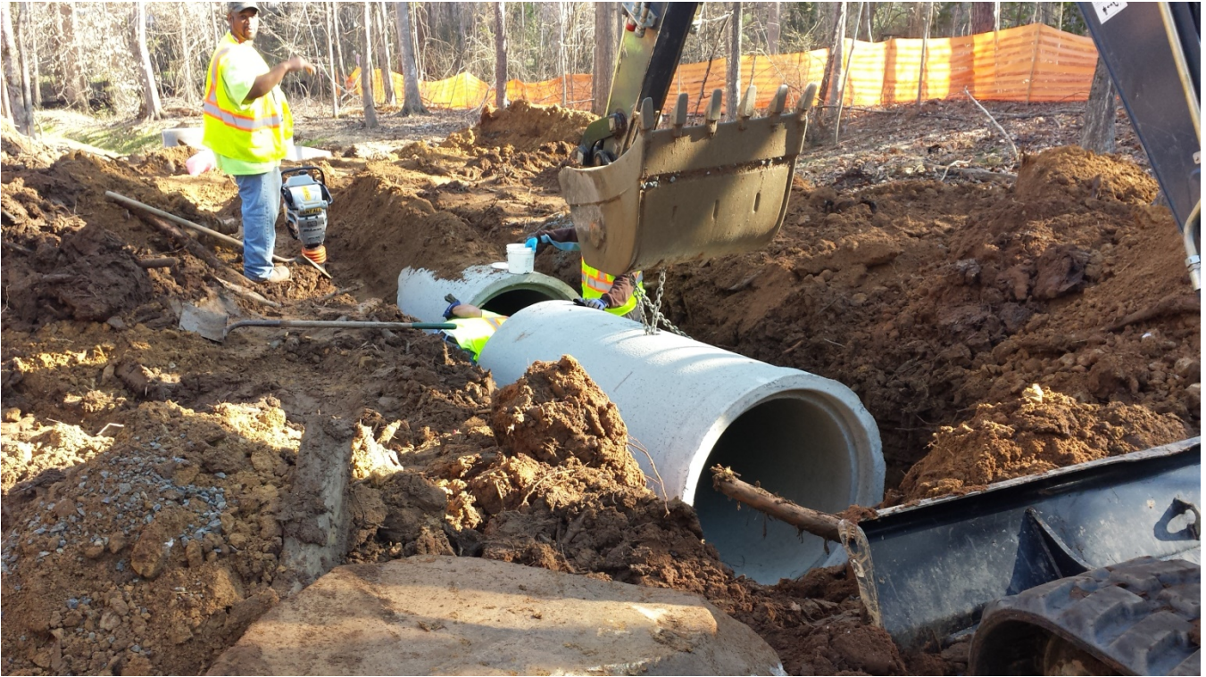
Photo 1: New concreted pipe installation in progress.
