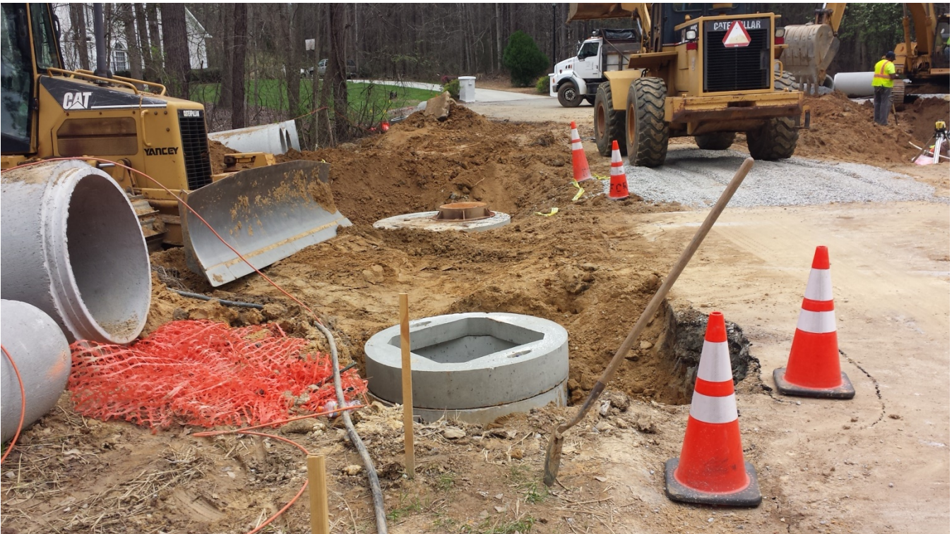
Photo 2: New drainage structures are being installed.
